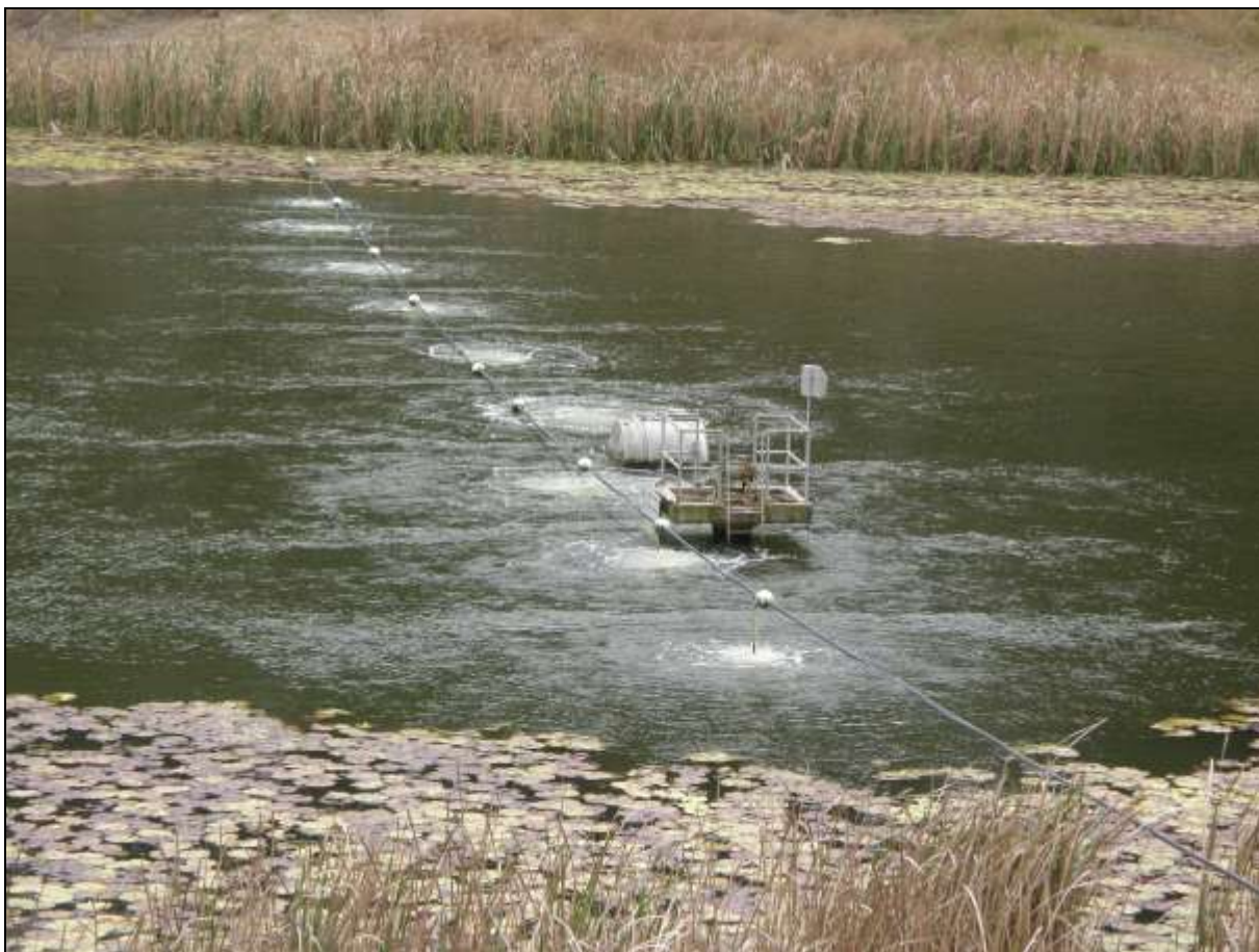
Aeration line suspended by stainless cable. Air stones set at various depths to follow dam base.
