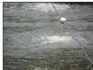
Aeration line suspended by stainless cable. Air stones set at various depths to follow dam base.
